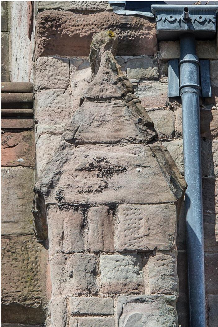
The friable nature of the stone revealed itself in flaking masonry and general decay and in 1907 was rendered to prevent further deterioration with what was initially thought to be 'Metallic Cement'.
